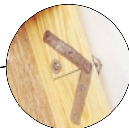
Metal hinges riveted on both sides of rail joints prevent side to side movement
